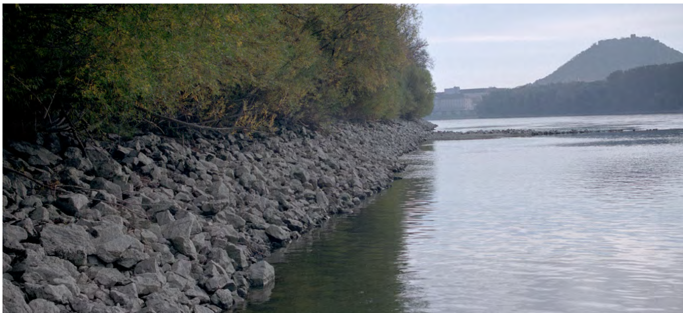
Riprap along the banks that was removed during the riverbank restoration, in Thurnhaußen, Danube River, Austria
