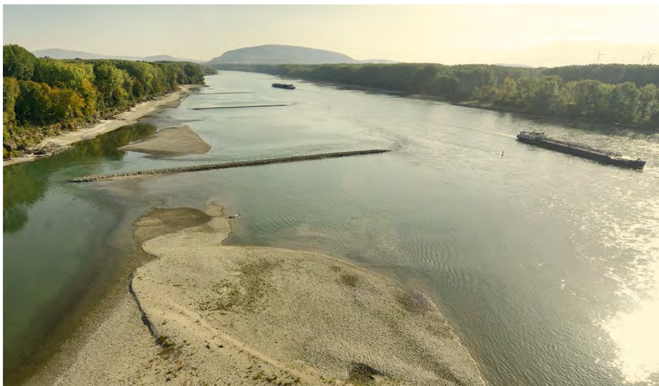
Groynes are innovative low-water regulation structures that allow fish migration. They are not connected to the Danube riverbank and are oriented downstream, to promote natural erosion, in Witzelsdorf, Austria. Photo: viadonau/Zinner
