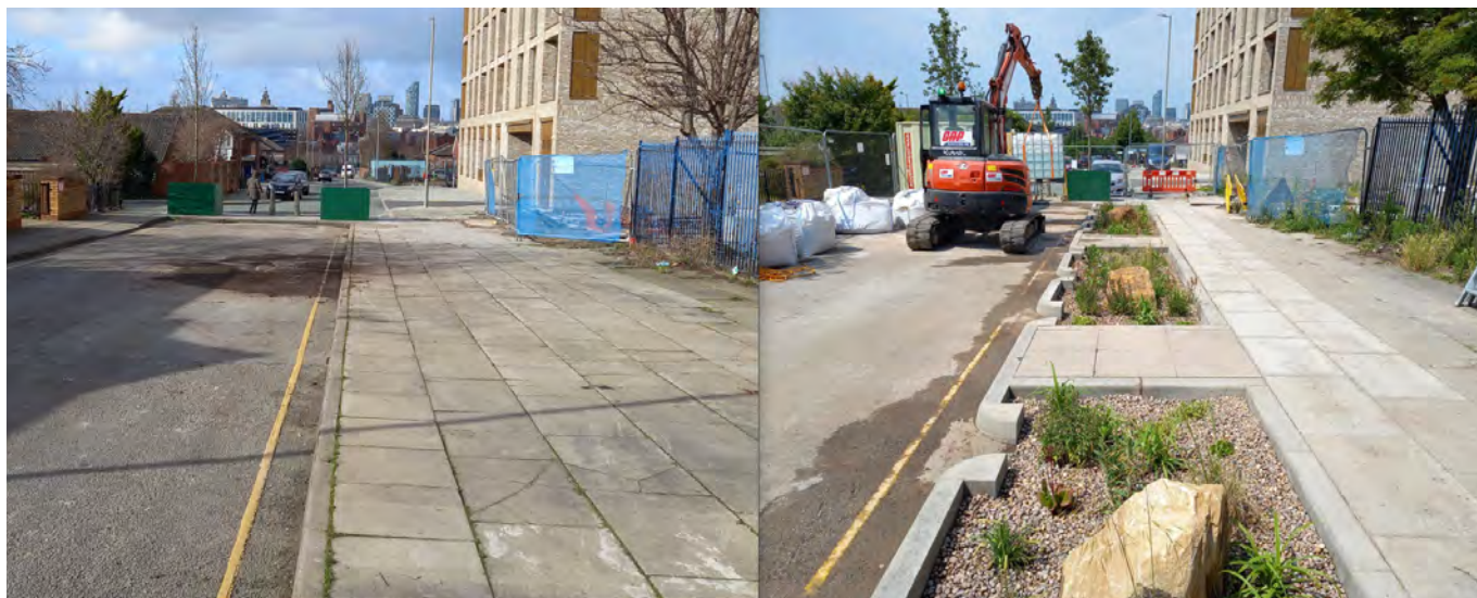
Before and after: Completed urban rain garden location at Upper Pitt Street, in Liverpool, UK Photo: STRI Group Ltd.
