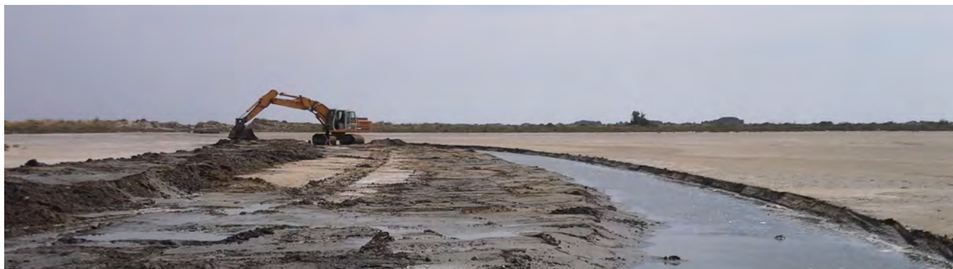
Channel dredging operation implemented as part of the hydraulic reconnection programme of Camargue former saltworks Photo: Parc naturel régional de Camargue
