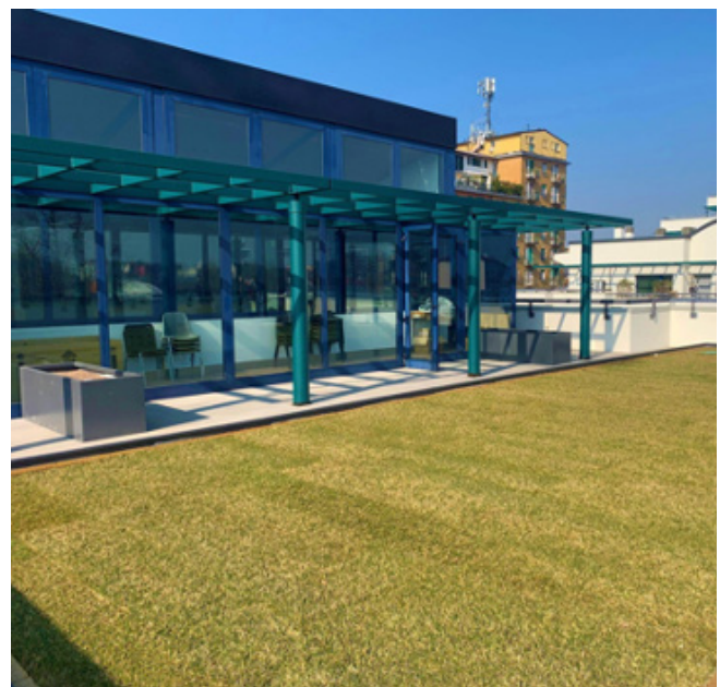
Green roof in E. Ponti (© Municipality of Milan)
