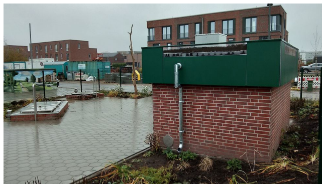
Smart blue-green roof in Hamburg (© BA Harburg)
