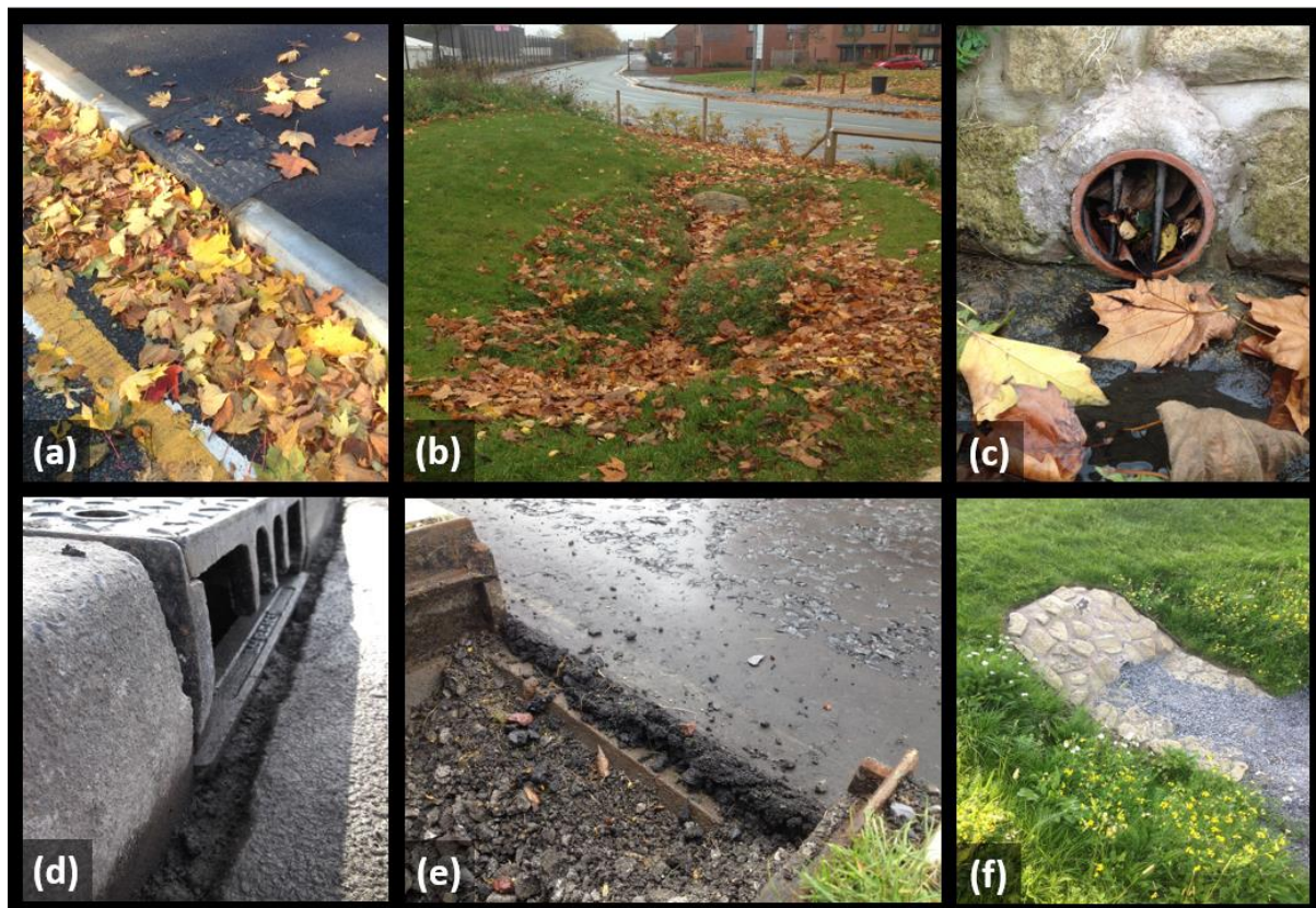
Figure 45. Park B Swale - leaves in the inlet (a), in the swale bottom (b), and in the pipework (c). Missing road material in front of Park A swale inlet (d), road debris following highway resurfacing works in the inlet of Park C swale, and slate chippings deliberately used to block headwall inlet in Park C swale (f). Photo credits: Professor Rothwell
