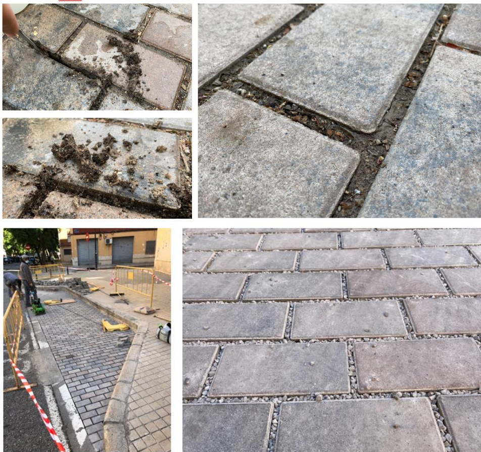
Figure 38 Blue Green Corridor - Foc Street SUDS Remedial Works
