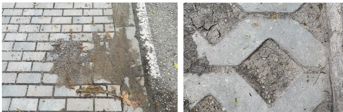
Figure 39 Blue Green Corridor - Foc Street SUDS showing sediment deposits
