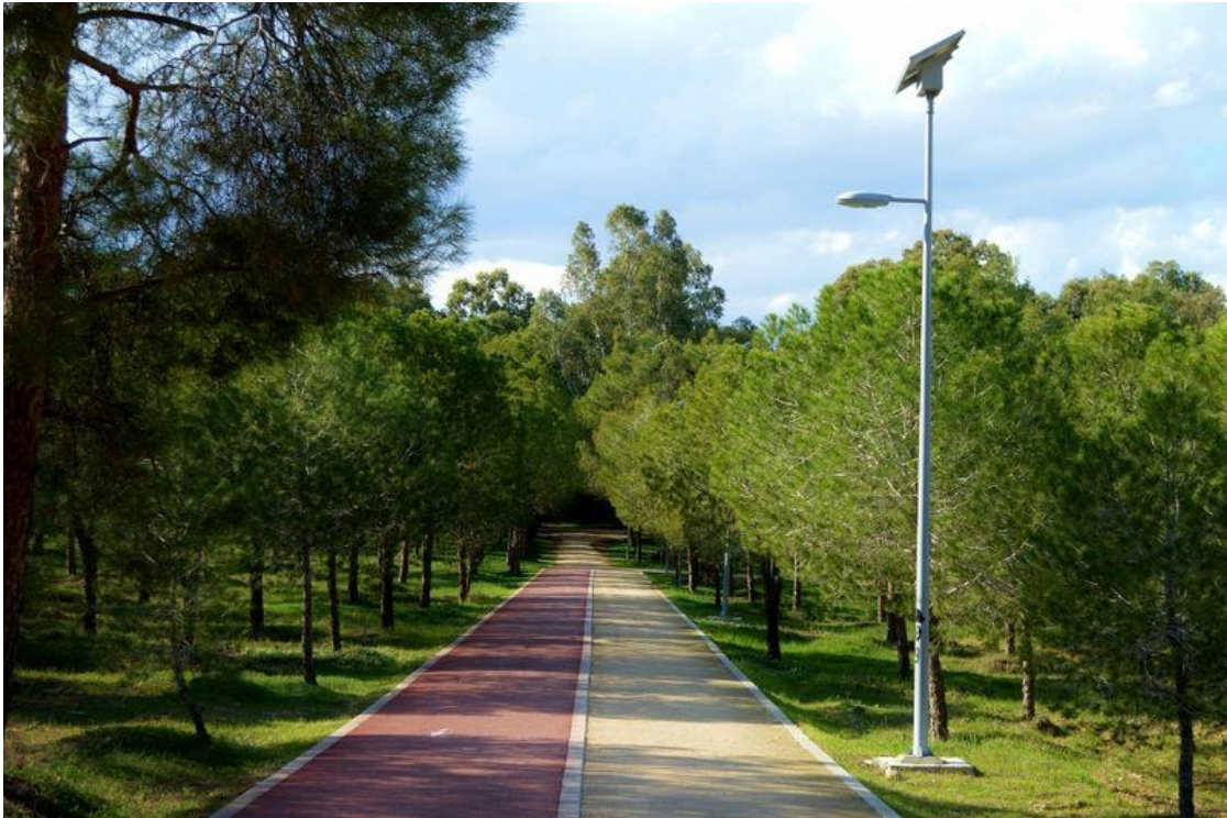
Figure 35: Improvements on the walking and cycling paths, solar panels installation (lighting)
