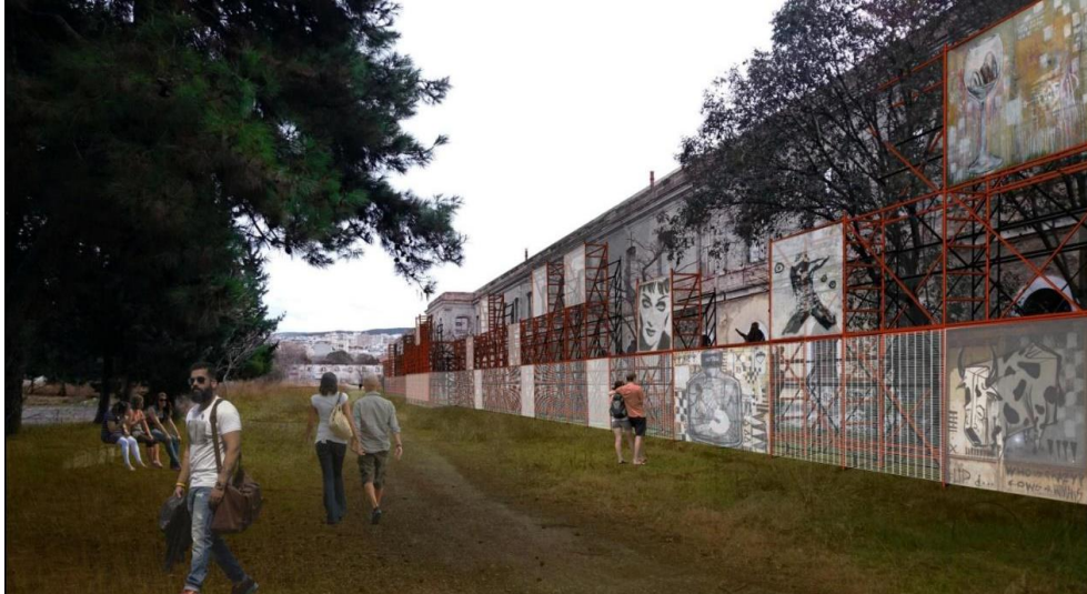
Figure * Protection scaffold of building
