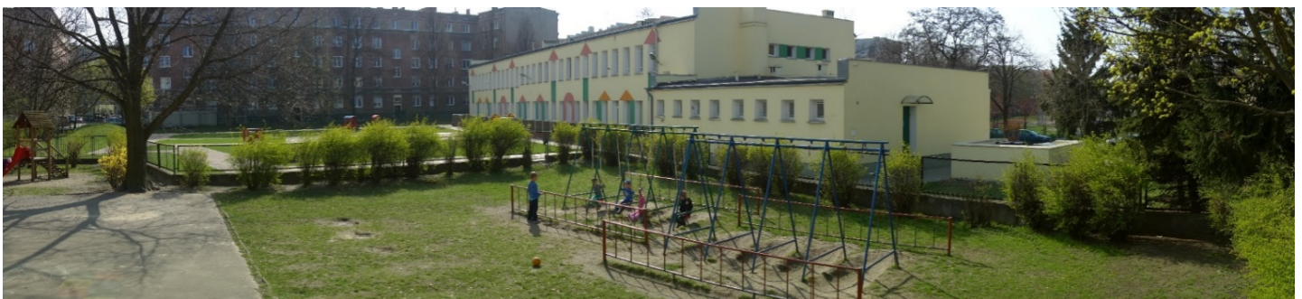
Pic. no. 3 The open garden before the work (April, 2017).
