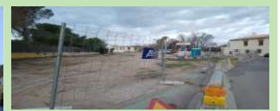
Construction phase in the degraded plot
