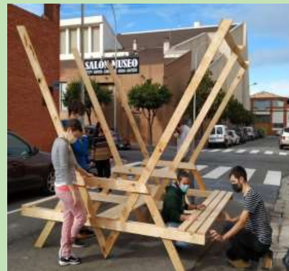
The students of carpentry and fallas art participating in it's construction
