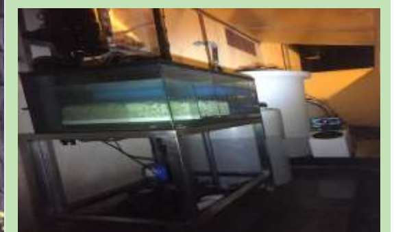
Water depuration system inside the shcool
