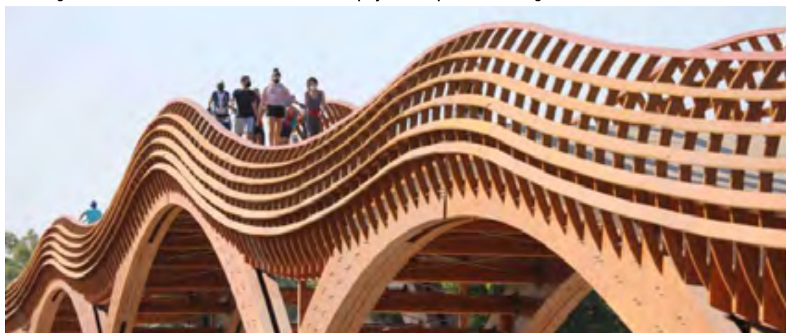
New bridge over Guadalhorce river. Part of the Senda Litoral project in the province of Málaga.
