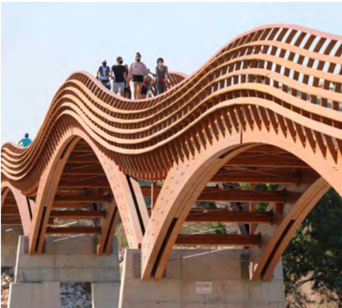
New bridge over Guadalhorce river. Part of the Senda Litoral project in the province of Málaga. Image source: http://www.sendalitoral.es/es/
